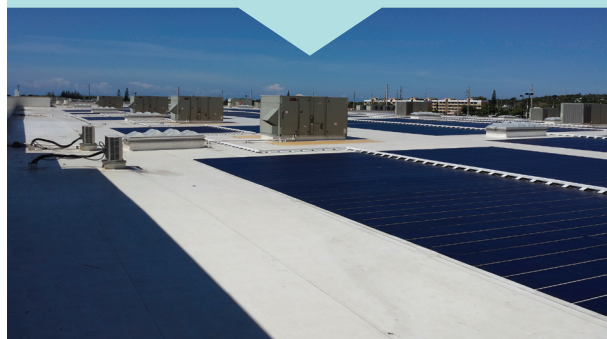
ONE OF FIVE TOSHIBA SOLAR ENERGY PROJECTS IN MASSACHUSETTS
